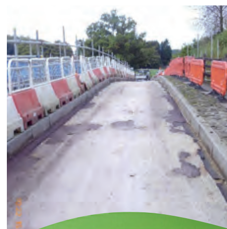
Carriageway Removal and Stone Removal
